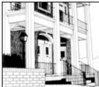
24-inch columns support a second story porch.
